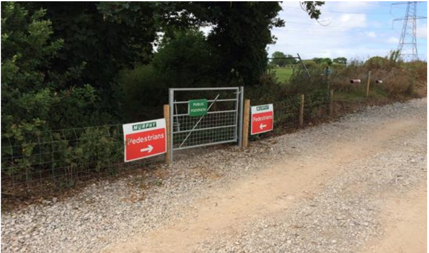
Figure 4.2: Example of managed crossing of a PRoW.
